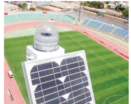
With minimal access for maintenance, stadium operators in Cyprus now enjoy hassle-free operation of AV23 units, installed as solar obstruction lights.
