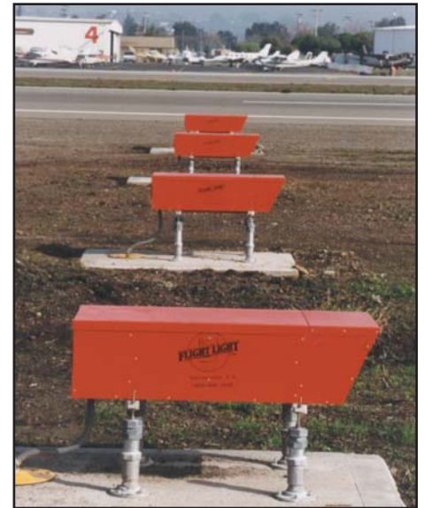
A 4-LHA installation. Four legs equipped with frangible floor flanges provide extra stability.
