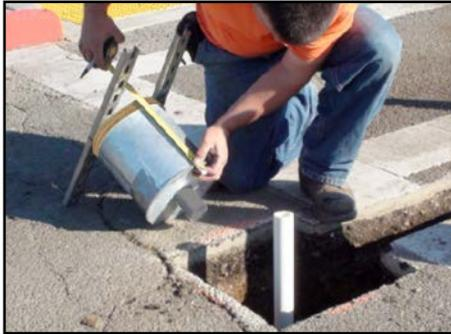
*Mounting Jig Attached to Base Can*
